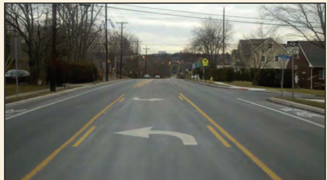
Ratzer Road (CR 705)- After Complete Streets Improvements Township of Wayne
