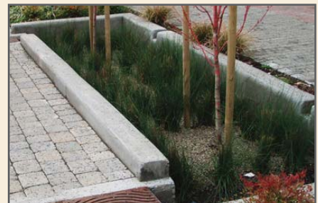
Infiltration stormwater planter with curb cut Philadelphia, PA Photo courtesy of Philadelphia Water Department
