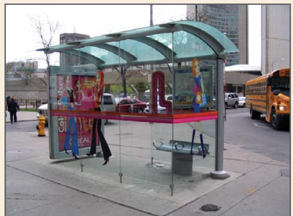
Bus shelters promote mass transit connectivity and provide an avenue to incorporate distinctive design elements of a Downtown Photo courtesy of Mike's Transit Stop
