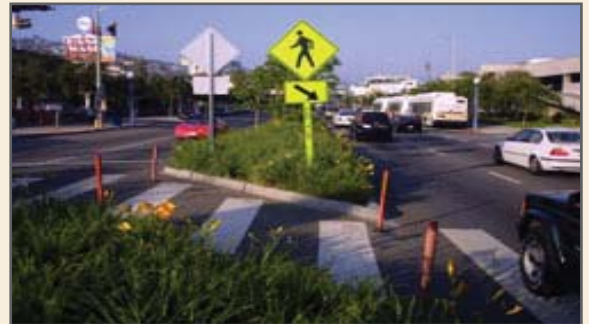
Crosswalk markings and pedestrian refuges provide safer environments for pedestrians at intersections Photo courtesy of Los Angeles County Bike Coalition
