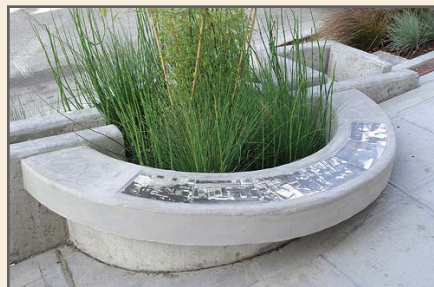
Flow-through stormwater planter with street bench Seattle, WA Photo courtesy of SvR Design Company
