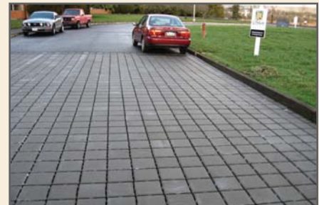
Interlocking pavers in parking area Photo courtesy of US EPA
