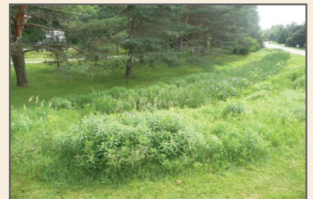
Bioswale, Bloomfield, MI Photo courtesy of Lawrence Tech College of Engineering
