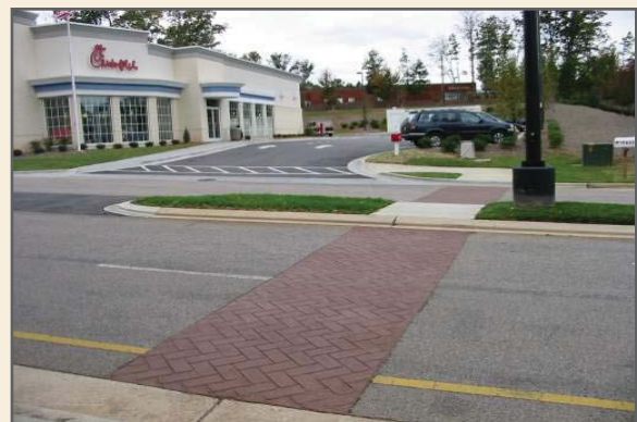
Medians provide an opportunity to beautify roadways and add safety measures, such as pedestrian refuges
