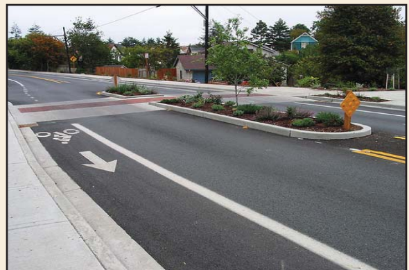
Medians provide safety for pedestrians and motorists as well as a place for streetscaping features such as plantings Photo courtesy of Richard Drdul
