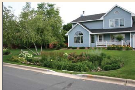
Curb Inlet, Burnsville, MN Photo courtesy of US Environmental Protection Agency c/o City of Burnsville and Barr Engineering
