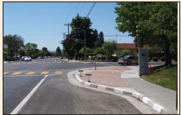
Curb extensions and chokers are two techniques that can be used to promote traffic-calming along a Downtown Street Photos courtesy of Richard Drdul
