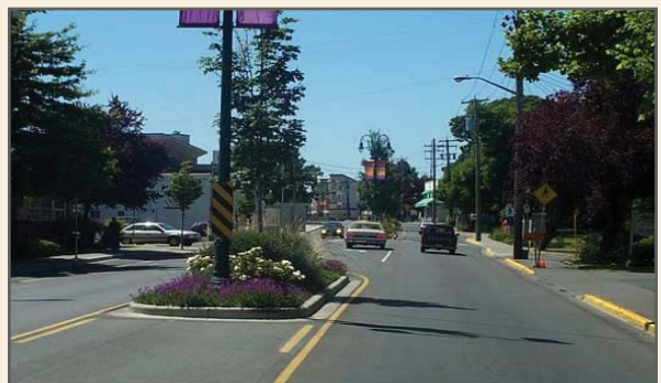
Medians can also be used to protect turning movements on busy roadways and allow easier flow-through traffic
