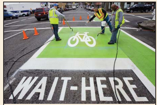
A bike box provides an area for bicyclists to jump ahead of cars when stopped at signalized intersections. This allows for safer interaction between vehicles and bicyclists
