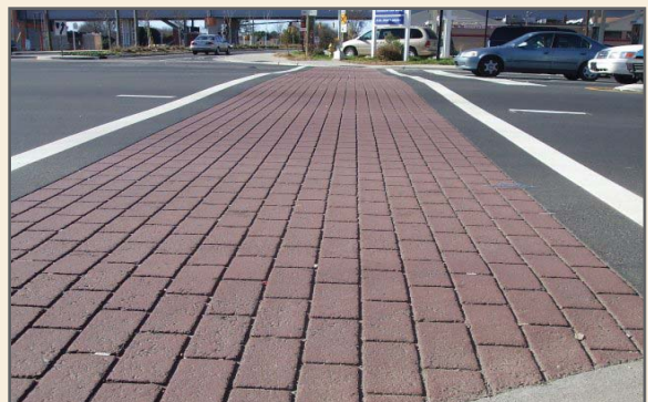
Pedestrian crosswalks can be marked in various patterns but they need to be highly visible to approaching motorists Photo courtesy of Pattern Paving Products
