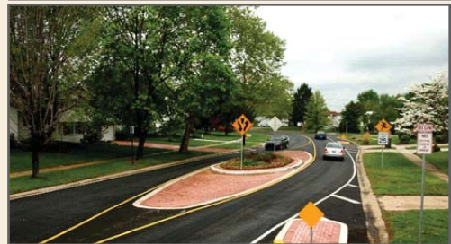
Curb extensions and deflector islands provide enough space to install bus shelters, green space and narrow intersection crossings
