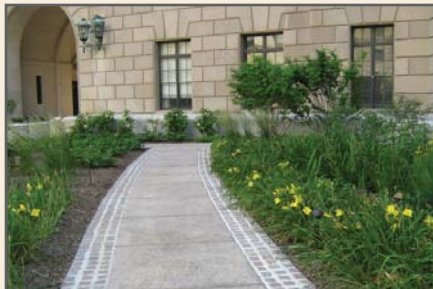
Pervious concrete walkway Washington, DC Photo courtesy of US EPA
