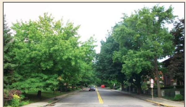
Street trees are a critical feature along any roadway and should be included in the beginning of any design process Photo courtesy of Local Ecologist
