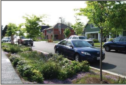
Grouped plantings in a bioswale Photo courtesy of US Environmental Protection Agency
