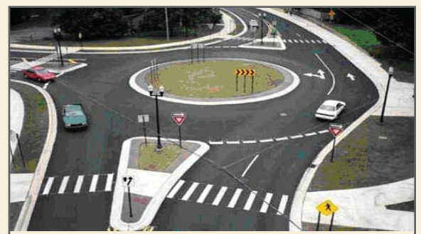
Medians can be used to organize traffic flows at major intersections or roundabouts Photo courtesy of Ingham County Road Commission
