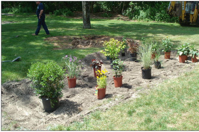
Plant layout for a rain garden in North Haledon as part of the Molly Ann Brook Watershed Management Plan.
