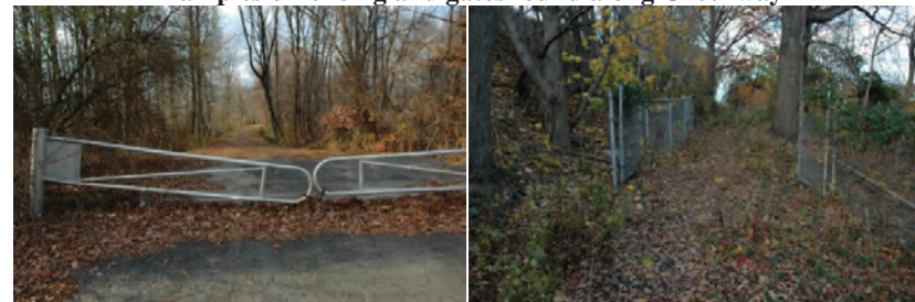
Picture left: North Jersey District Water Supply Commission gates near West Belt Parkway Picture right: Woodland Park Department of Public Works gates near Rose Place
