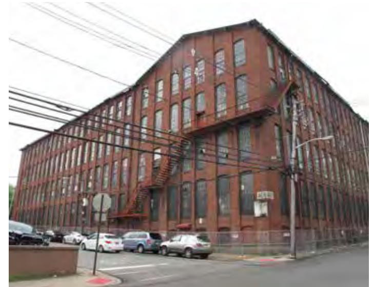
Miesch Mill, adjoining the park entrance on Jasper Street, is eligible for the National Register.
