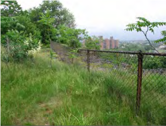
Issue: Visitors will be drawn to the cliff edge to take in the views, posing a safety hazard that must be mitigated by a secure yet attractive barrier.
