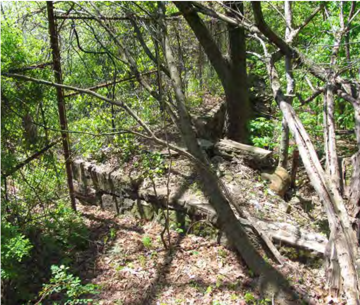
Ruins of the Middle Reservoir wall, showing corner seen in historic image on page 56. (photo: G. Archimede)
