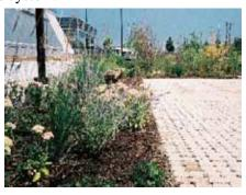
**Vegetated Swales** – a broad, vegetated channel used for the movement and temporary storage of runoff. Swales planted with native vegetation are effective in reducing the volume, rate, and pollution potential of runoff.
