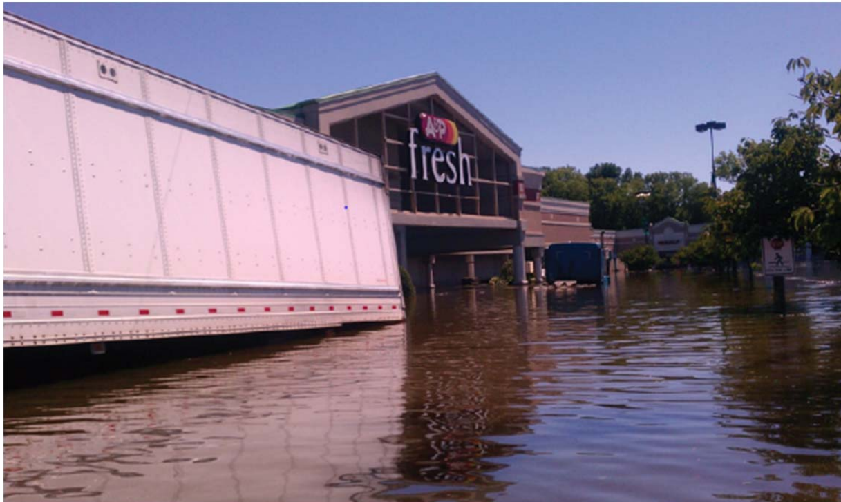
Pompton Plains, NJ (Photograph by John J. Trainor, US Geological Survey).
