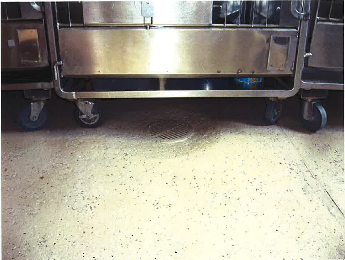
Photograph 5: A floor drain present in the cat building.
