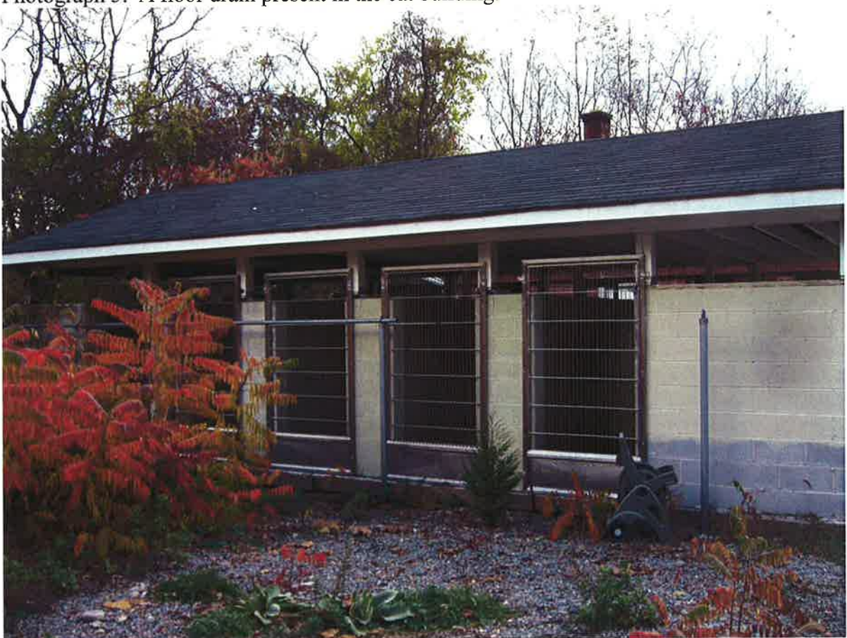
Photograph 6: View of the western side of the structure containing five (5) kennels.
