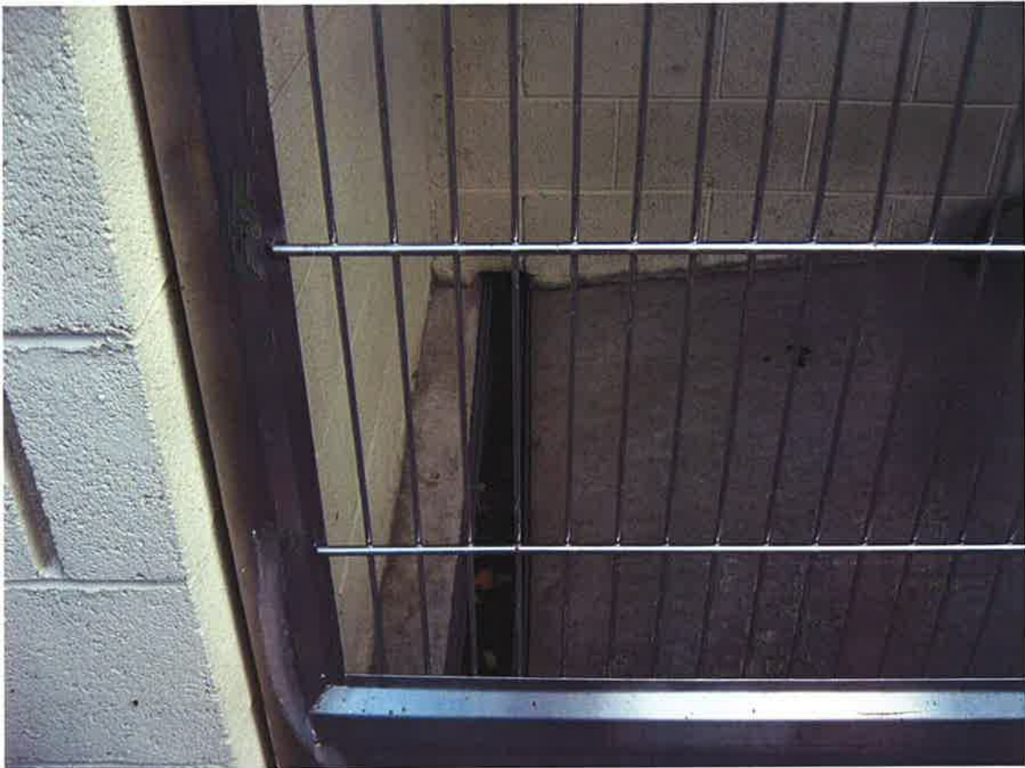
Photograph 13: Drainage provided in each of the five (5) kennels.
