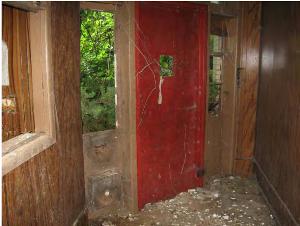
Front Office Entrance
