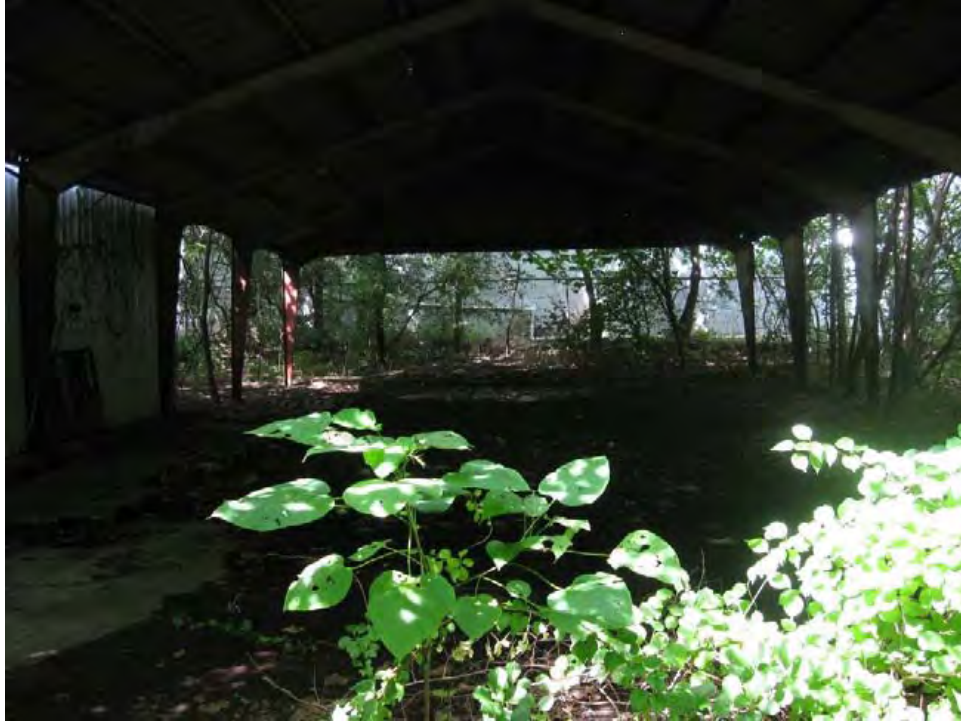
Solvent Storage Canopy
