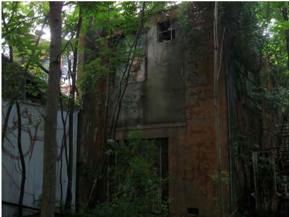
Rear of Area #5 and Solvent Room
