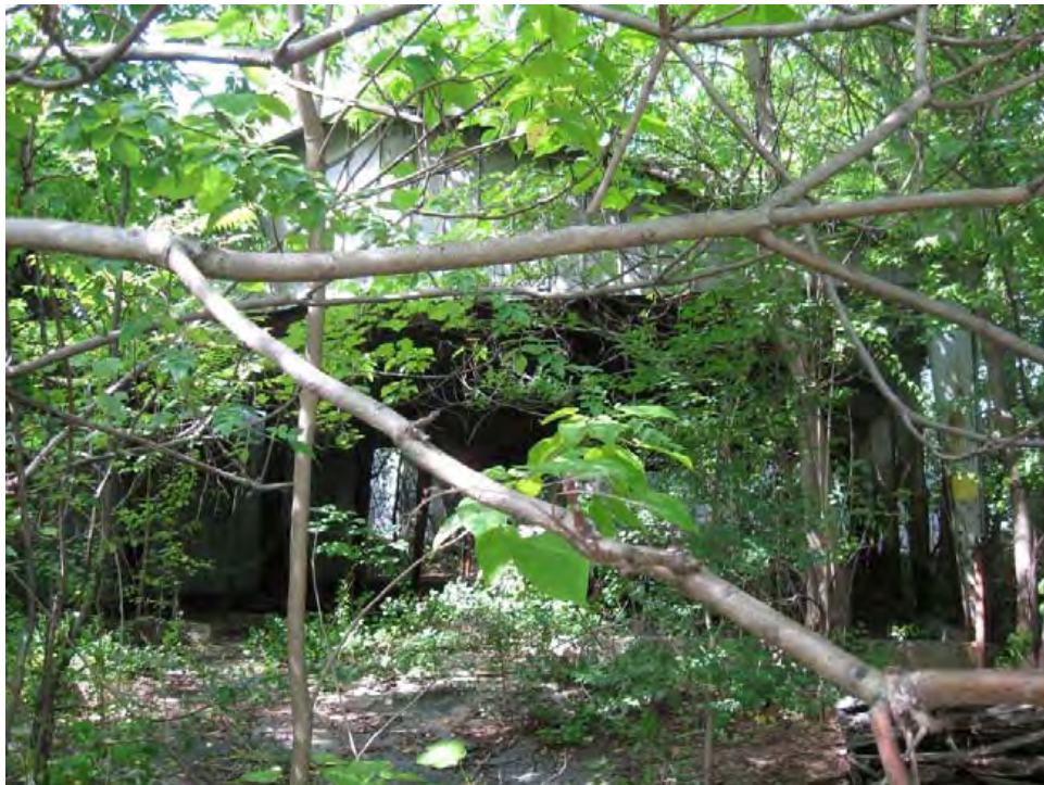
Solvent Storage Canopy
