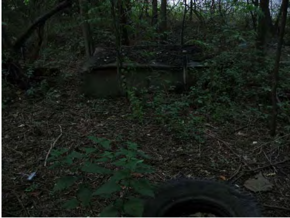
UST Gate Valve Control Chamber
