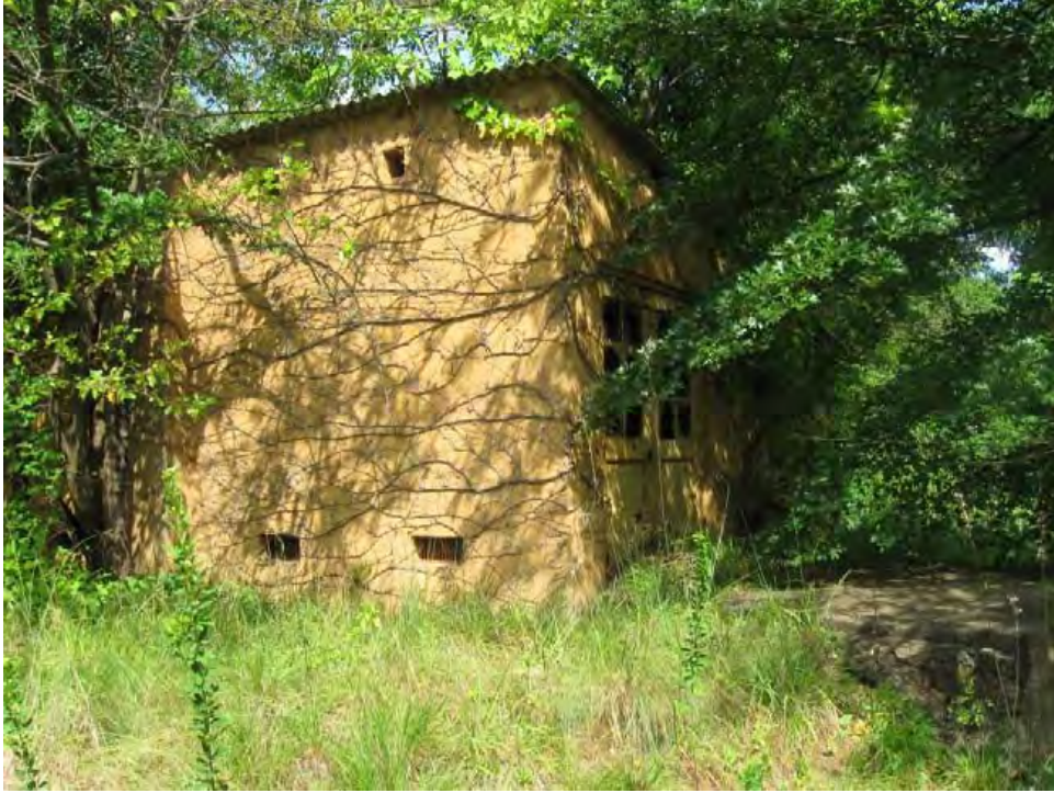
Nitrocellulose Storage Shed
